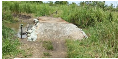
Figure 2Local bridge in Mambu Boma
